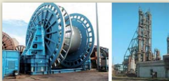
Decommissioning of industrial plants in Italy: Brindisi and Assemini (CA).
