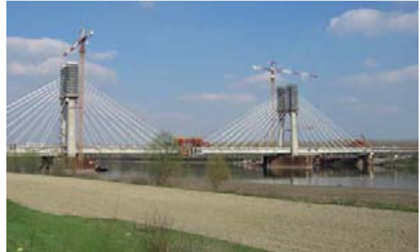
High speed rail track bridge on Po river
