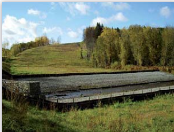
Situation after final reinstatement
