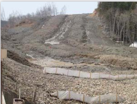
Situation after backfilling
